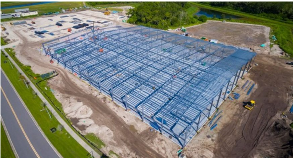
Figure 16. OneWeb's $85 Million Satellite Facility under Construction
